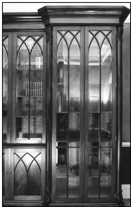
Fully adjustable saw-tooth shelf system with hand-turned and fluted columns and mahogany faced hoop pine shelves
